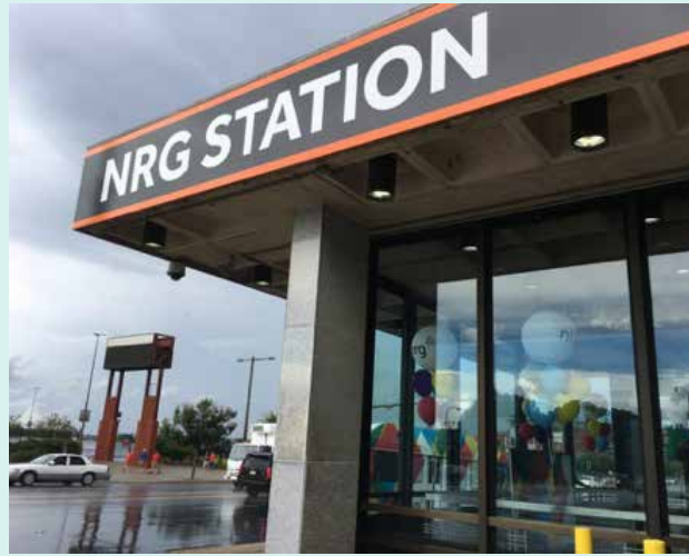
Figure 17: A view of NRG Station from the street.
