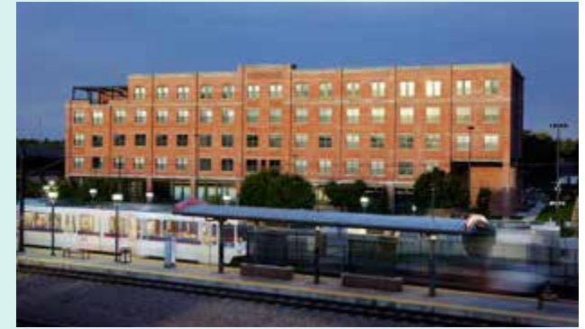
Figure 21: Evans Station Lofts, in Denver, CO. Denver TOD Fund purchased this one-acre parcel and developed this five-story workforce housing development—the first ever family-based low-income housing to be build adjacent to a Denver light rail station.
